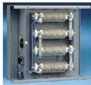
External resistance bank used for larger-horsepower motors
